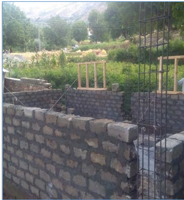
Construction of Computer Lab for Girls College funded by Solas
